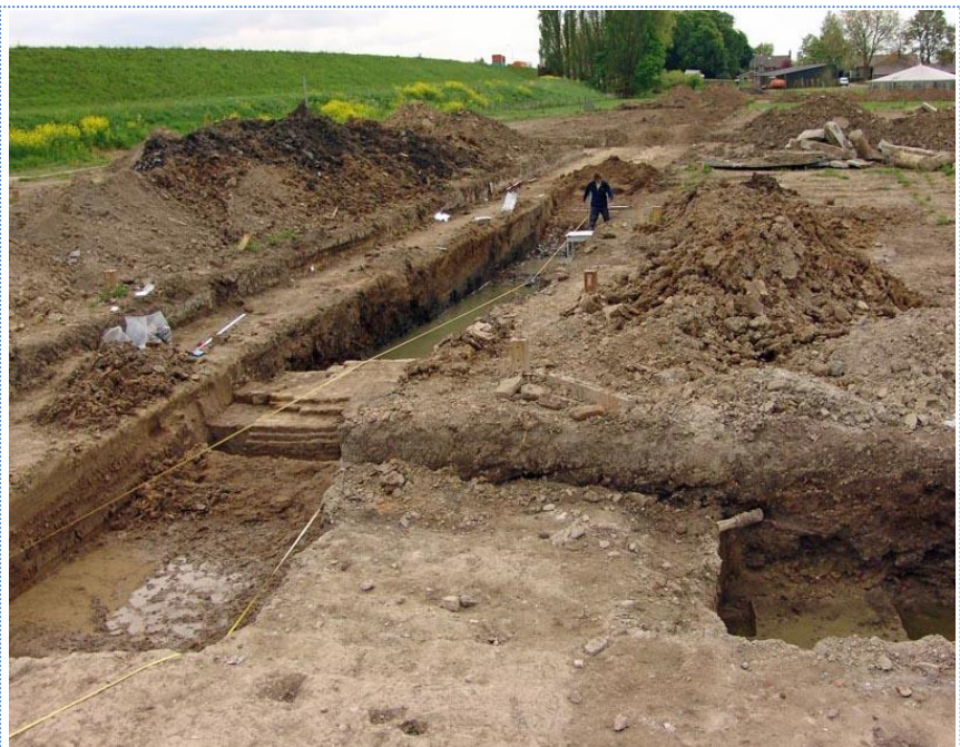
Excavations of the foundations of a 13th century tower of Het huys Varick. On the left side you see the dike that protect us from flooding
